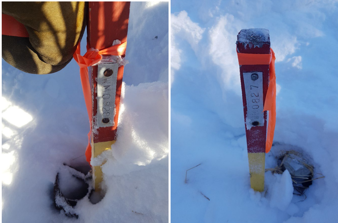
Figure 12-3. Collars for drill holes WM08-28 (left) damaged casing and WM08-27 (right).
