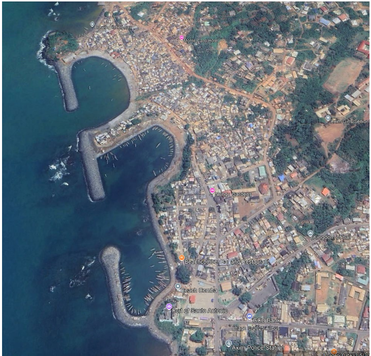
Figure 2-5: Aerial View of Axim Harbour #1 and #2
