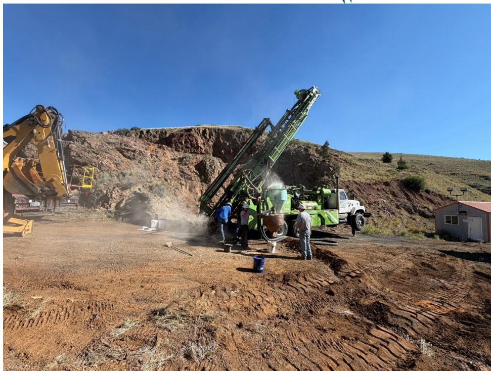
Image 1: O'Keefe Drilling testing the first RC hole (Hole ID M26RC-01)
