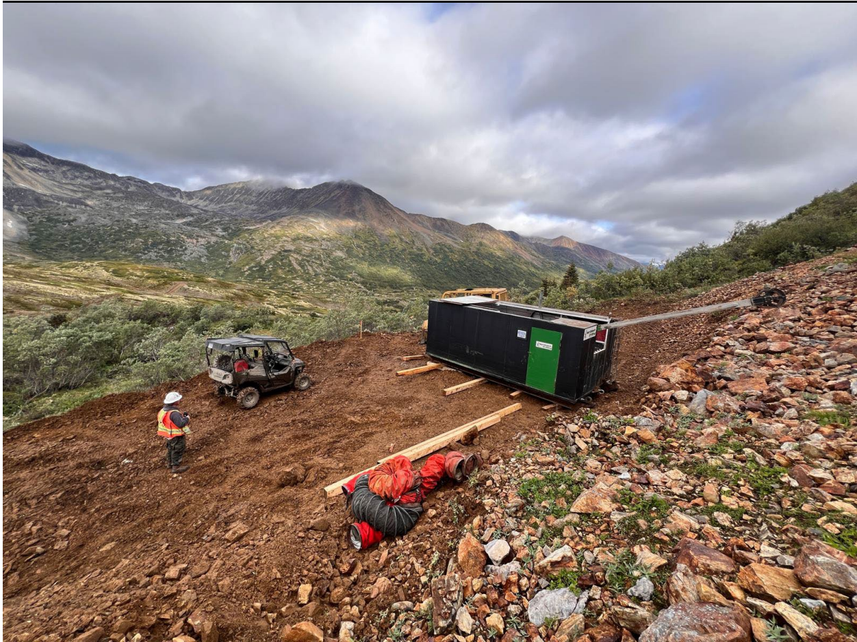
Figure 1: Drill pad final preparation for maiden drill hole on Kuhn target, Magno project
