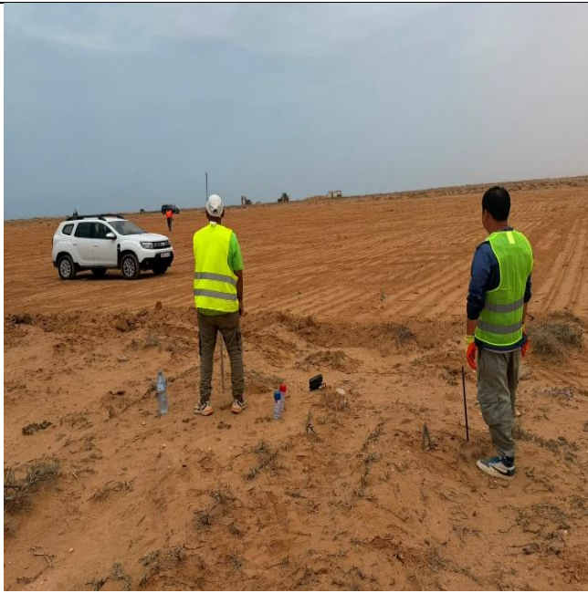
Surveyor's for Preparatory Work to get ready for the Pilot Plant TitanBeach Project facing West
