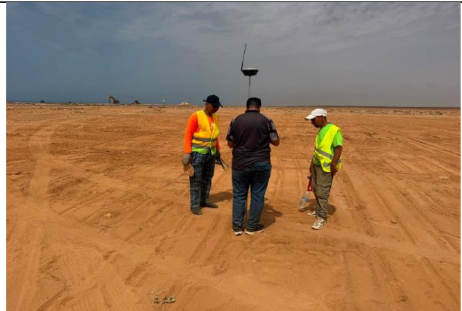
Surveyor's for Preparatory Work to get ready for the Pilot Plant TitanBeach Project facing West
