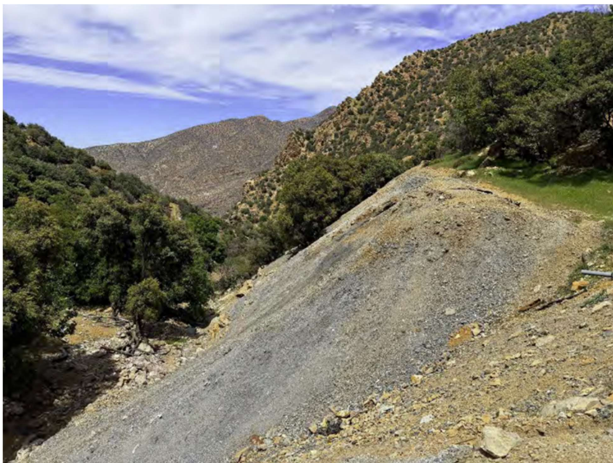
Figure 21: Trail built up with waste material for sample 31326.
